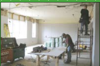
February 8, 2008 • Dry wall
